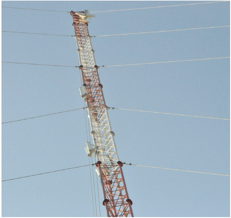
Network base station tower; with attached wireless antennas (right).
