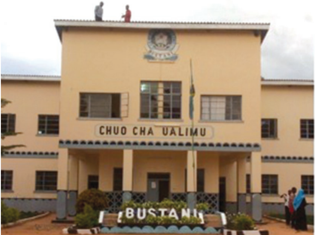
Technical team members from KCN install equipment at Bustani Teachers College in Kondo.
