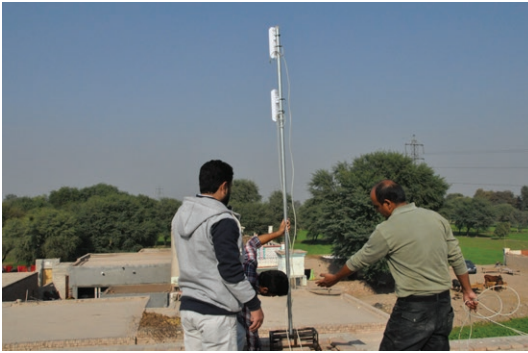
Team installing antenna for connecting the village.
